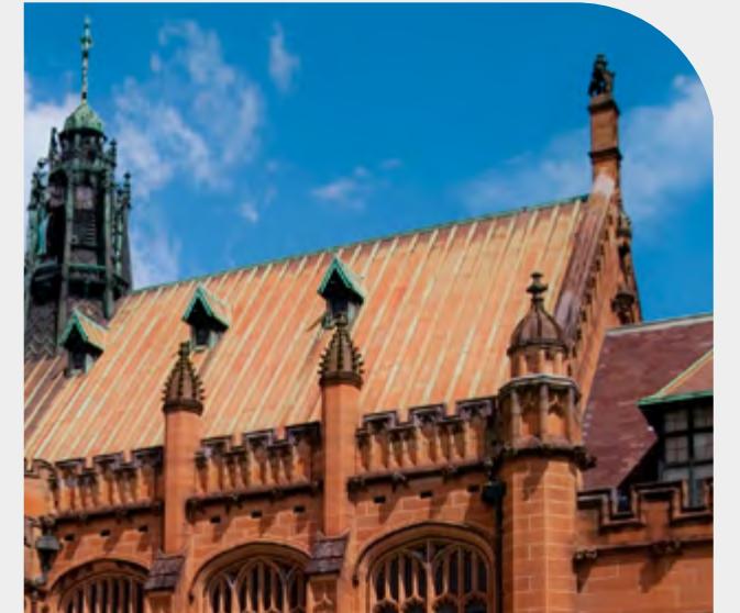
The University of Sydney, building detail
